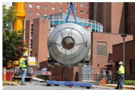
Magnet weighing 38,000 pounds lifts off from South Drive
