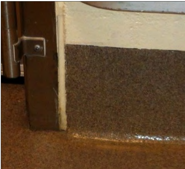
Figure 4.4.4.2.2 Integral Cove Base Detail
