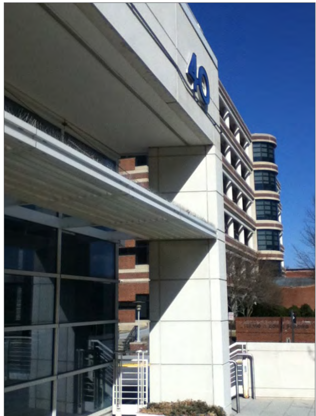
Figure 4.1.6 Sunshading at Building Entrance
