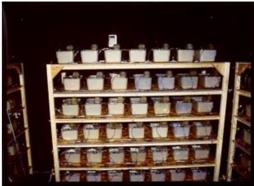
Figure 5.3.06 Typical Rack: Populated Room
