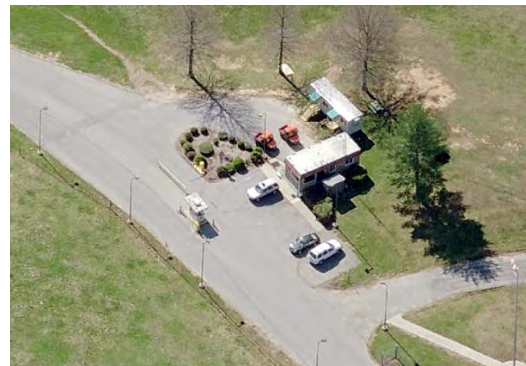
Building 115, the Original Security Building and the Replacement Trailer Looking East
