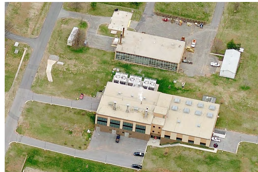
The Original and the Current Central Utility Plants Looking North
