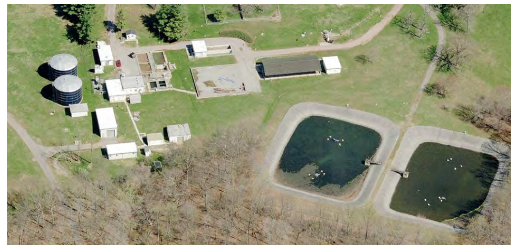
The Wastewater Treatment Plant (WTP) Area Looking North
