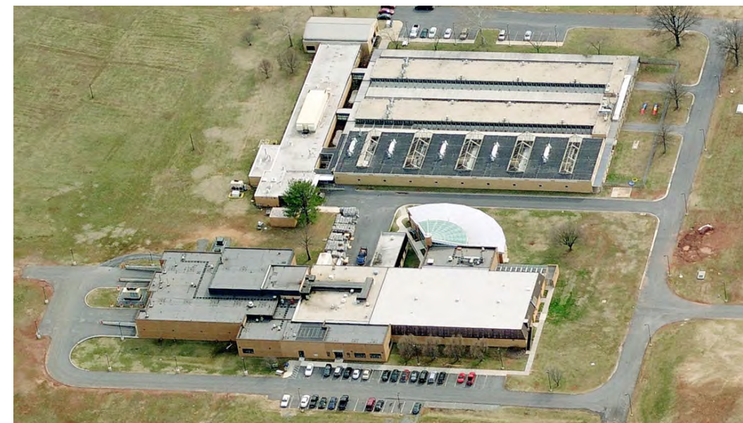
Buildings 103 and 102, Looking South
