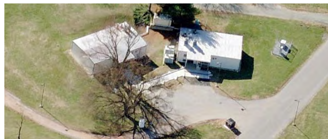
Buildings 127 and 128, Looking West.
