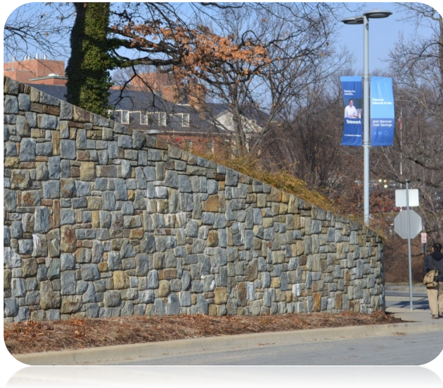
Exhibit 6.4.A. Typical Campus Retaining Wall
