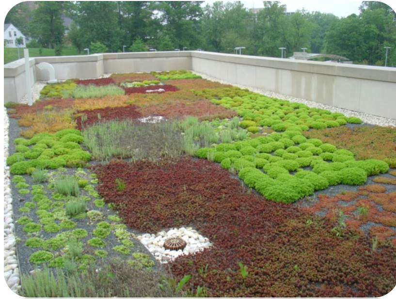
Exhibit 6.4.O. NIH Bethesda Gateway Center Green Roof
