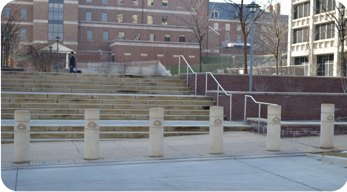
Exhibit 6.4.N. Precast Concrete Type Bollard with NIH Logo Example
