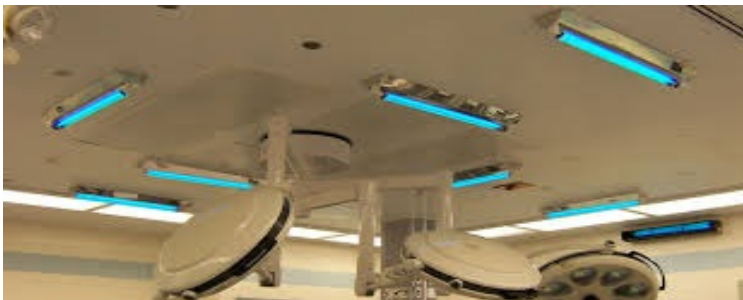
Figure 1 – Downward UVGI Lamps
