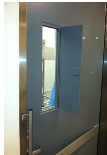
Figure 2: Light-tight cover on lab door.
