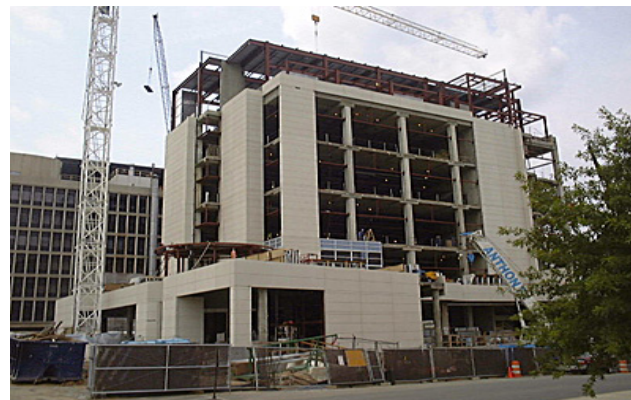
Figure 1: Concrete structure and finish panels
