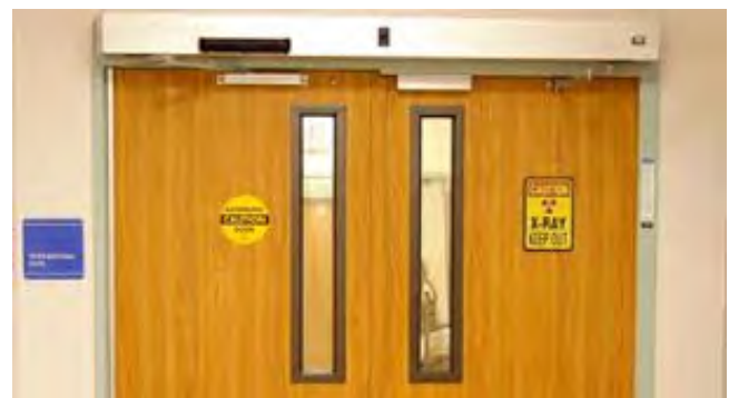
Figure 4.2.4: Lead-lined shielded doors, windows, and door frames
