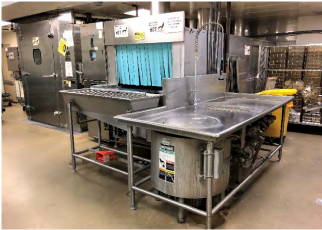
Figure 2.4.5.6.E: Cage wash with waste disposal system
