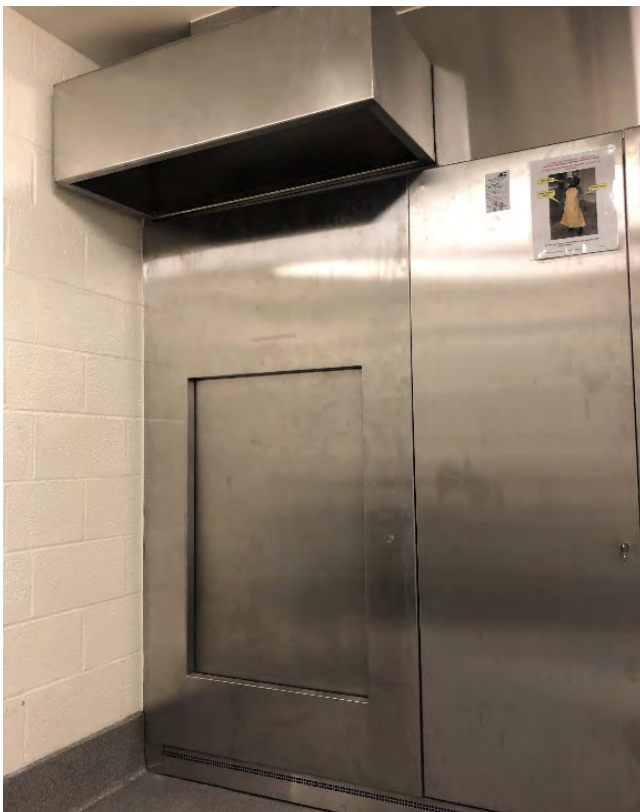
Figure 2.4.5.6.F: Capture hood over an autoclave
