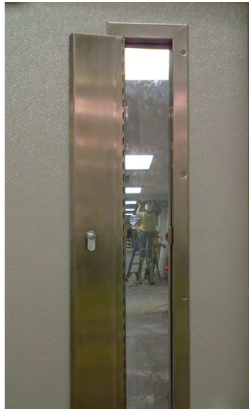
Figure 4.2.2.7: Vision panel with hinged cover
