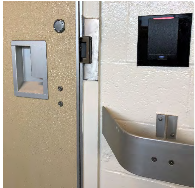
Figure 2.4.4.D: Card reader and electro-magnetic lock (Credit: NIH OD/ORS/Division of Veterinary Resources)
