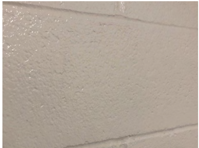
Figure 4.3.3.3.C.2: Epoxy paint with no pinholes (Credit: NIH OD/ORS/Division of Veterinary Resources)
