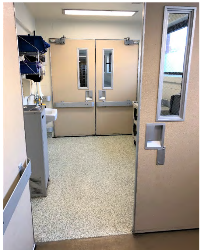
Figure 2.3.2.3: Anteroom with FRP doors with view windows, handwash sink, and PPE storage (Credit: NIH OD/ORS/Division of Veterinary Resources)
