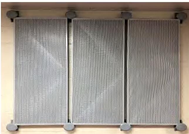
Figure 2.4.5.15: Sound attenuation panels (Credit: NIH OD/ORS/Division of Veterinary Resources)
