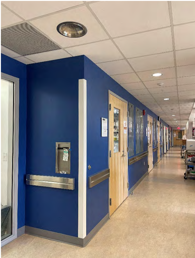
Figure 2.2.5: Open lab corridor with safety shower
