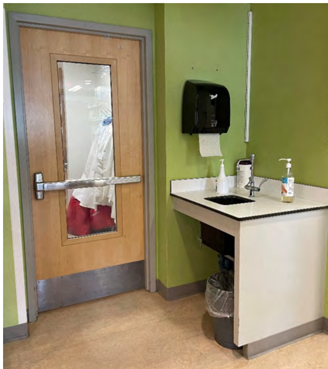
Figure 2.2.3.B: Handwashing sink at exit
