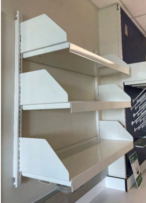
Figure 4.5.1.3: Max. shelving support spacing – 3 ft.
