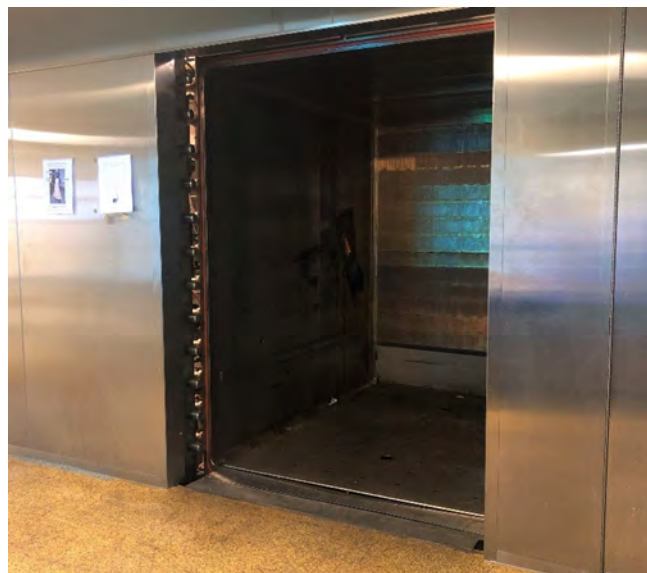
Figure 2.3.1.2: Bulk sterilizer with stainless steel modular wall
