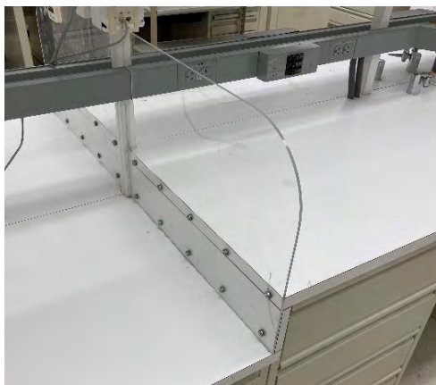
Figure 4.5.3.1.D: Splash guard between high and low bench example
