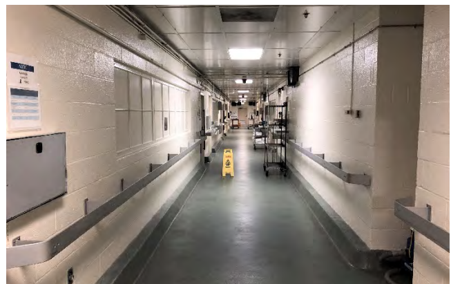
Figure 2.4.5.7: ARF corridor with integral base epoxy floor and wall protection
