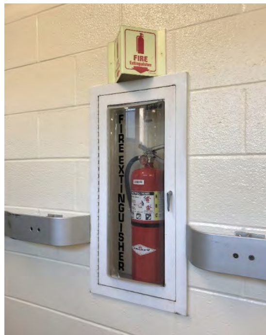
Figure 2.4.3.E: Wall protection at a fire extinguisher (Credit: NIH OD/ORS/Division of Veterinary Resources)
