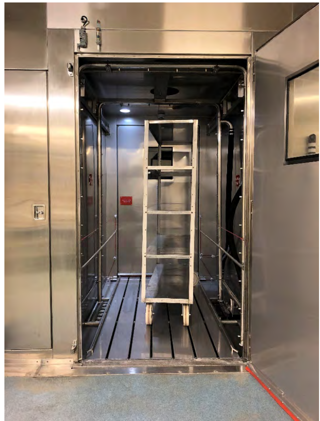
Figure 2.3.4.2.A: Rack cage washer (Credit: NIH/OD/ORS Division of Veterinary Resources)
