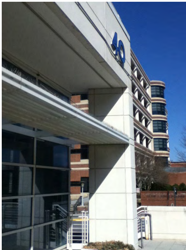
Figure 4.1.6: Sunshading at building entrance
