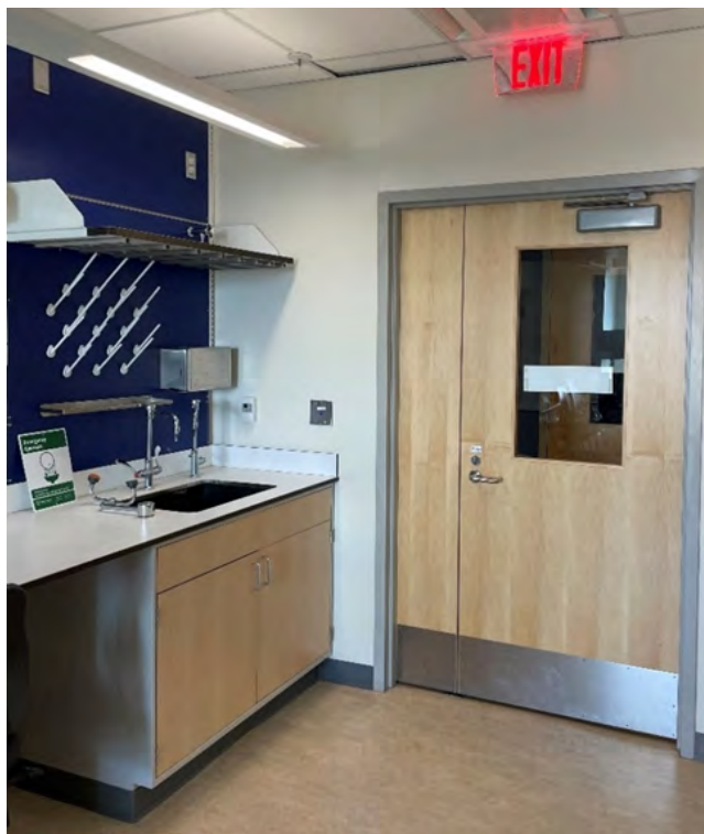
Figure 2.2.3.A: Laboratory sink also serving as a handwashing sink at an exit
