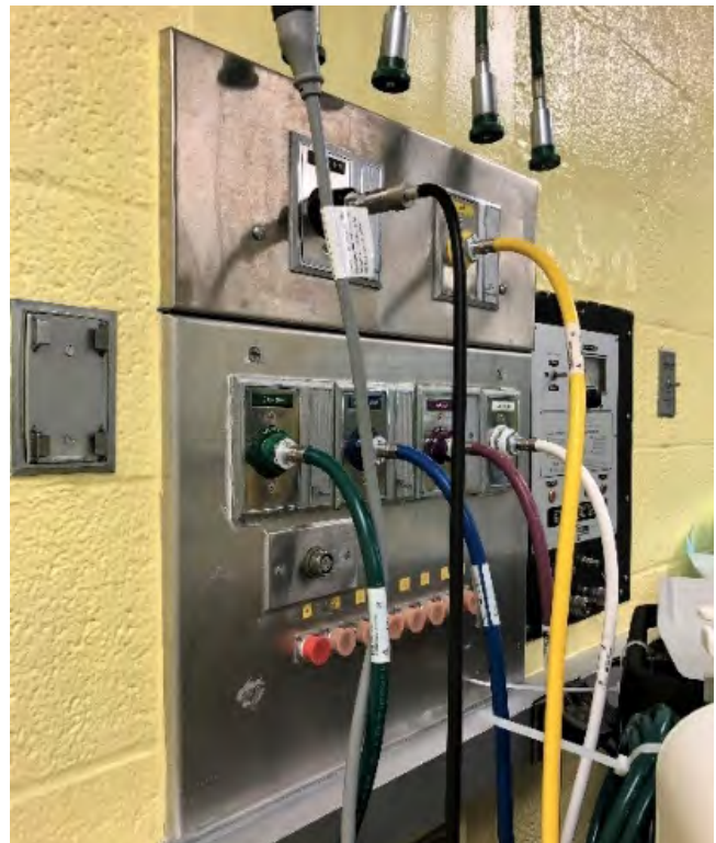
Figure 2.4.5.10.B: ARF surgical gas panel
